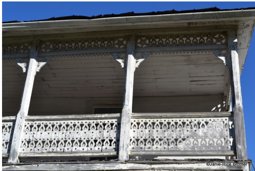
Figure 8: A detail of the intricate balustrade and frieze on the porch.
