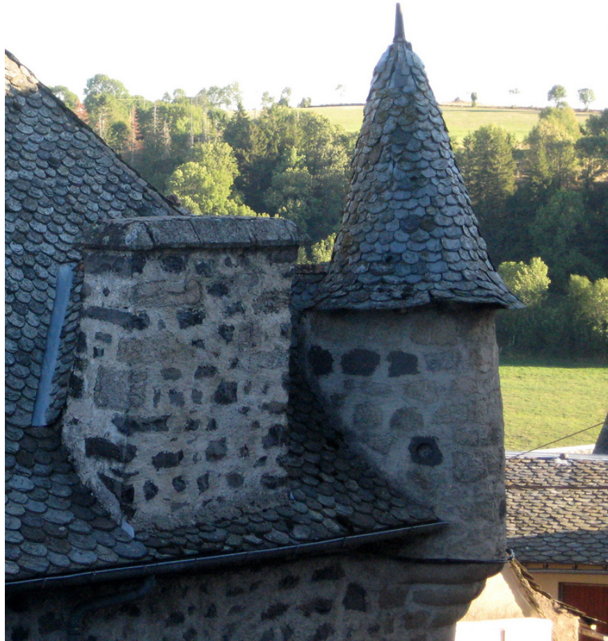
Figure 18: Lauze Tile Roofing - Auvergne,France
