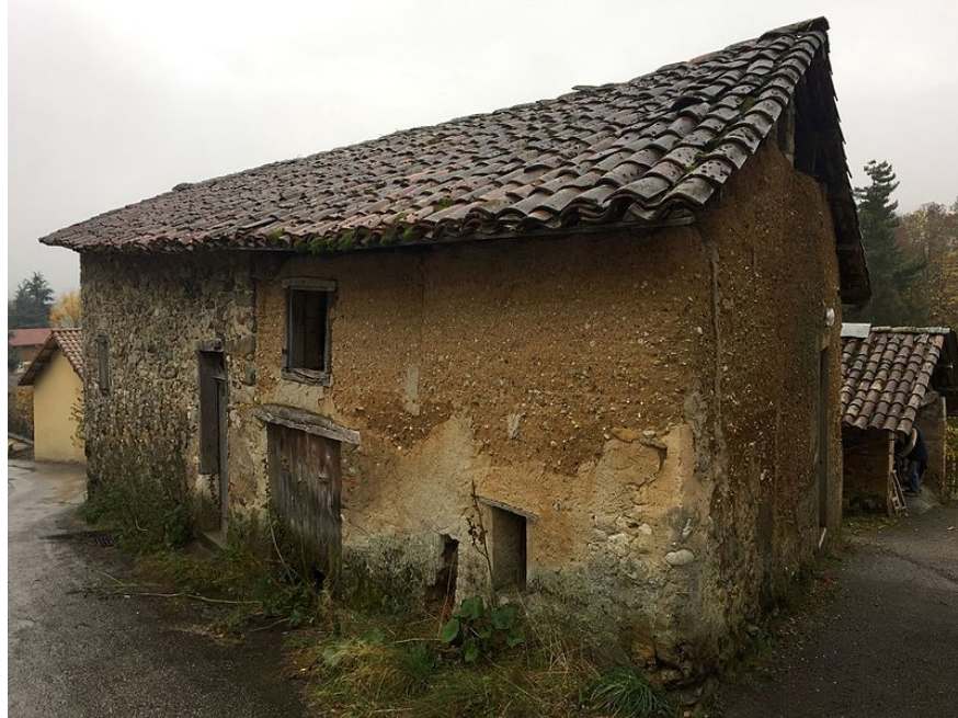
Figure 19: Rammed Earth (Pisé) Building - France
