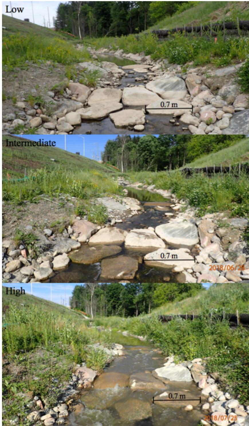
Figure 5. Looking upstream at VRW2 (a low gradient rock weir) under low (top photo), intermediate (middle photo), and high (bottom photo) water level conditions. It is evident that orifice flow is the only active flow regime under low water level conditions, while orifice, gap, and over-weir flow are active simultaneously
