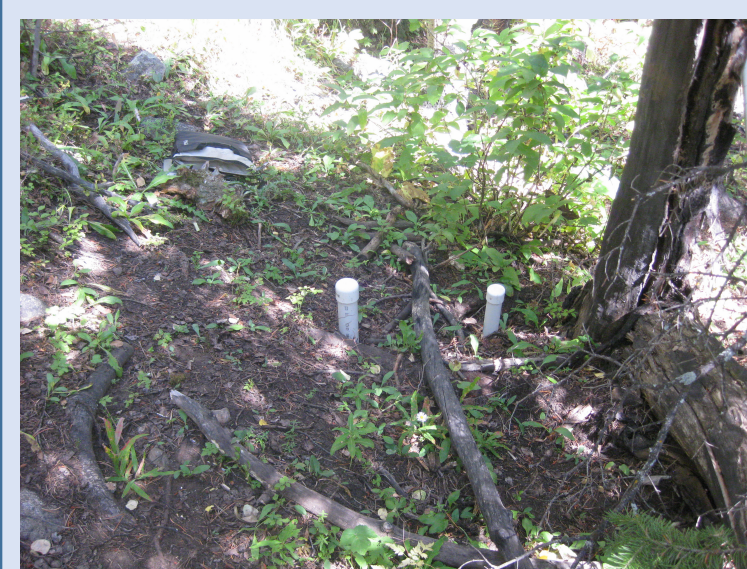
Fig 2. Groundwater wells were installed at each transect.
